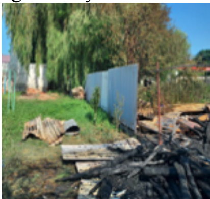
Photo of the fence damaged by the fire.
